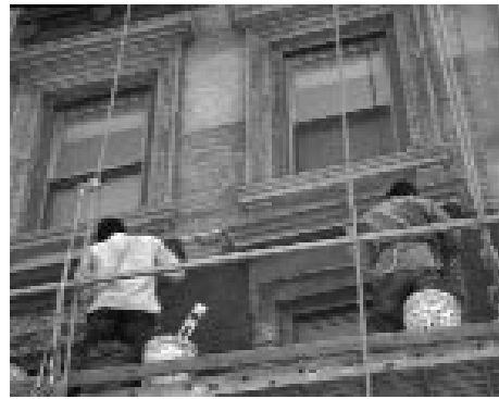
Years of weathering caused the brownstone details to deteriorate (left), but careful composite repairs (center) restore it to its original glory (right)
