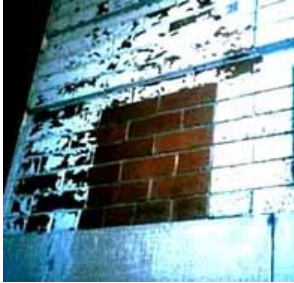
Any cleaning method should be tested before using it on historic masonry. Photo: NPS files.
