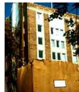
The lower floors of this historic brick and architectural terra-cotta building have been covered during chemical cleaning to protect pedestrians and vehicular traffic from
