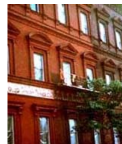
Appropriate cleaning of historic masonry. Photo: NPS files.
