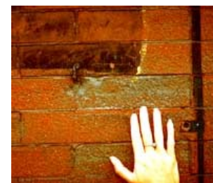
Undamaged historic brick (above). Sandblasted brick (below). Photo: Courtesy, Illinois Historic Preservation Agency.
