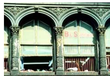
Cast iron may be abrasively cleaned, but must be painted immediately to prevent rust. Photo: NPS files.
