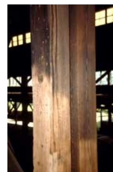
Industrial interiors that are not finely milled may be abrasively cleaned, in some instances. Photo: NPS files.
