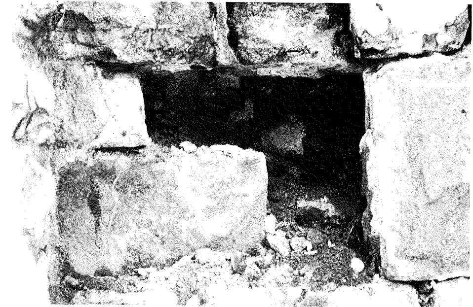
Mortar turned to sand by prolonged penetration of acid rain, St. Mary's Cathedral, Kingston, Ontario.
