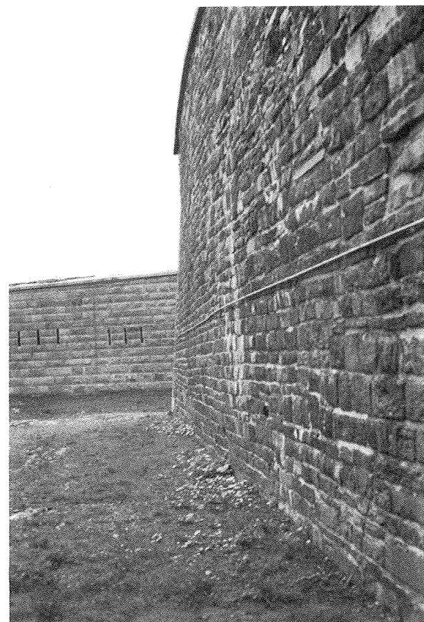
Bulging wall face caused by loss of internal mortar.
