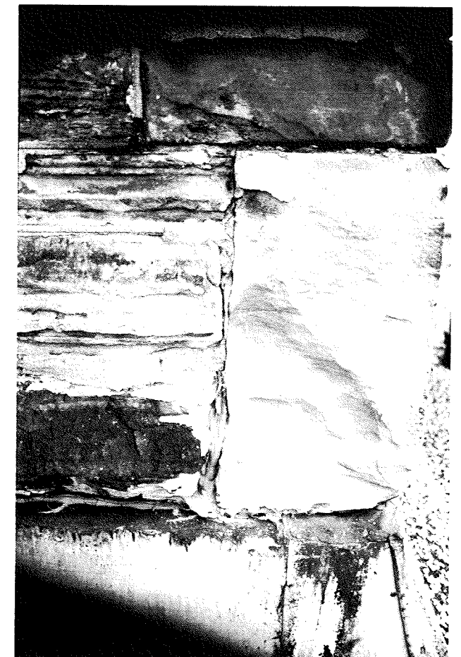
Two different types of sandstone weathering differently on the corner of a tower. The Ohio sandstone on the right is suffering from "alveolar erosion" caused by wind vortices and the increased deposition of water soluble salts caused by higher evaporation rates at the corner.
