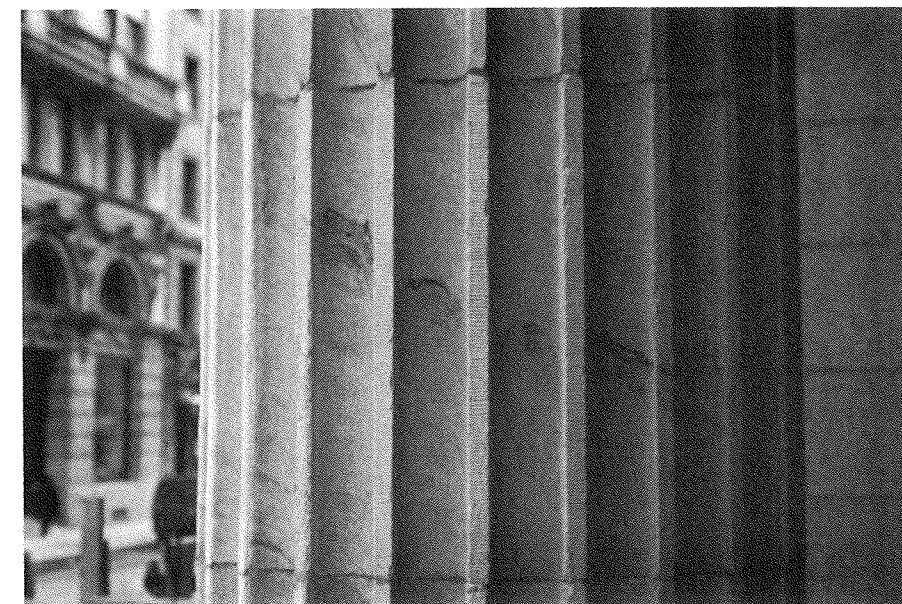
Acid soluble stone; note the damage to left face which was exposed to the rain.
