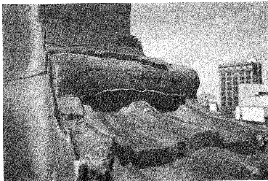
Contour scaling in red sandstone.
