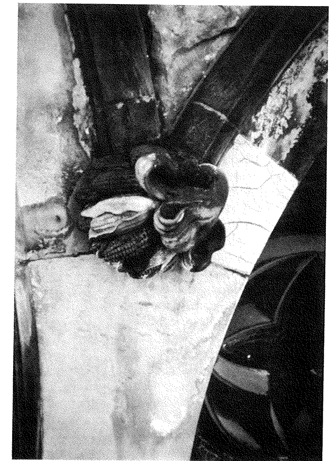
Poultice of diatomaceous earth and water being used to remove salts.
